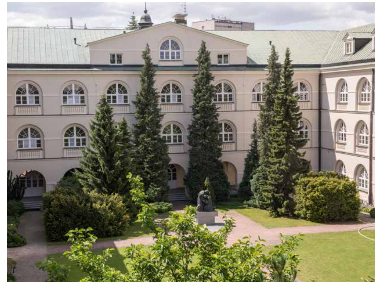
GG - MAIN BUILDING (Al. Racławickie 14)
